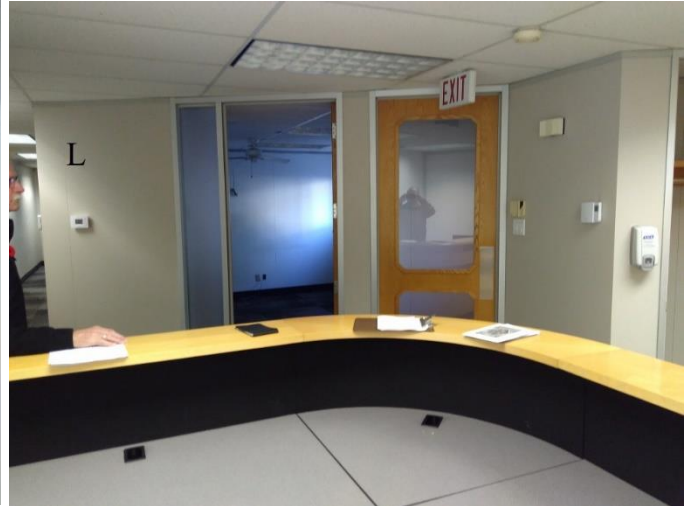
L: Another view of the studio entrance. The front entrance way is getting demolished.
